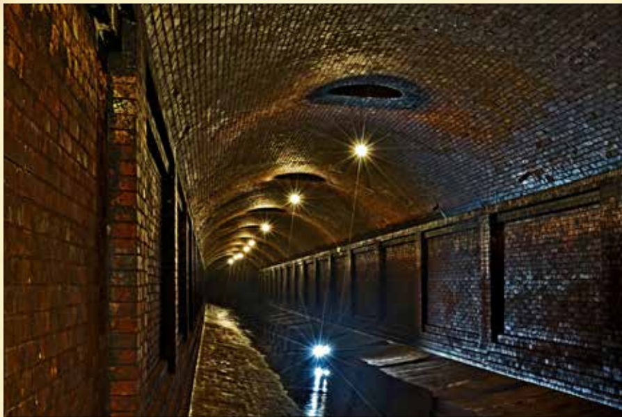
raw water sedimentation tanks
